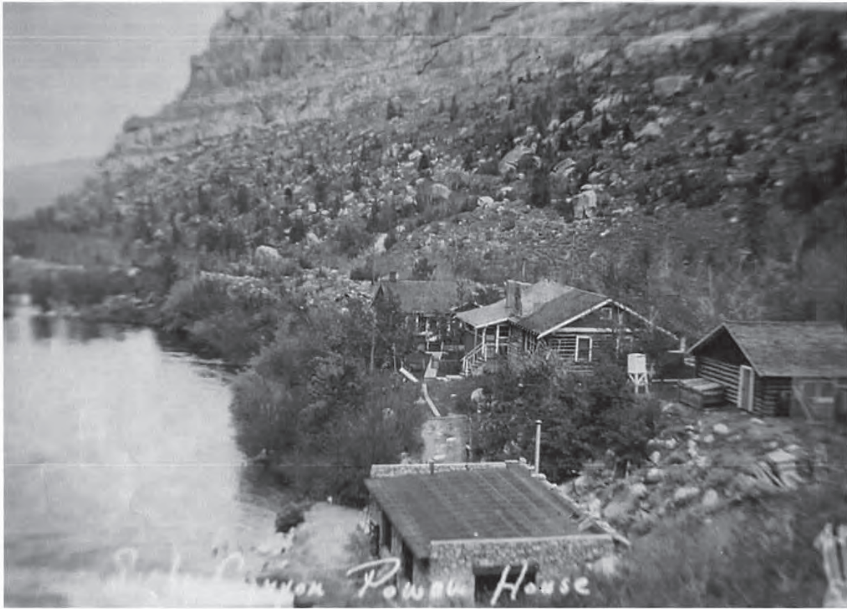
Sinks Canyon Power House, 1925
